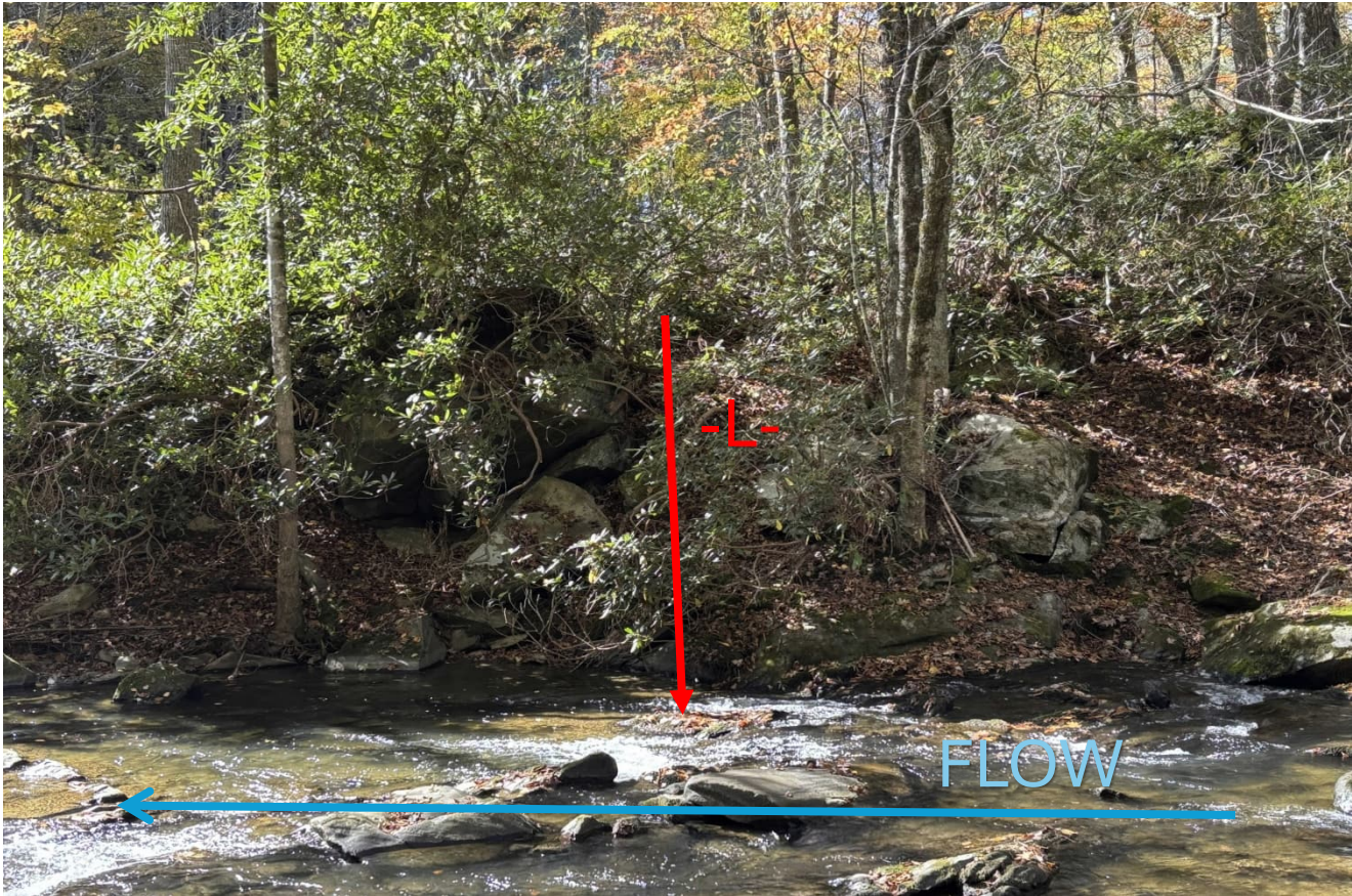
View to south from Bent 1 towards End Bent 1 showing boulders, rock outcrop in river and bank
